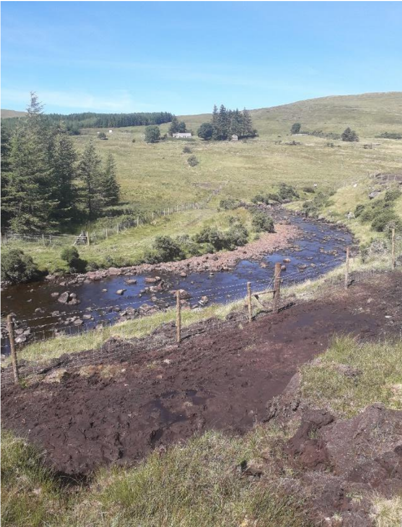
Figure 50: fencing implemented along the Reelan River.
