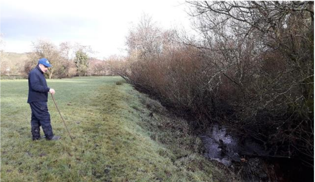
Figure 91. Before. Lack of fencing
