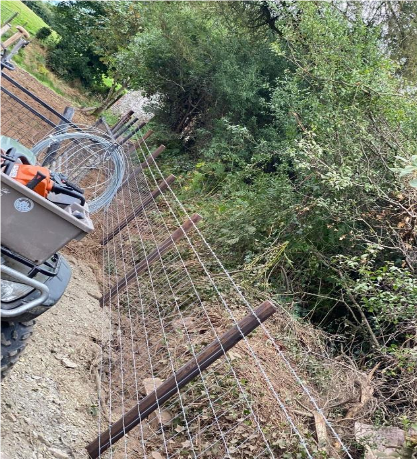
Figure 21: fencing erected along the recreational walkway of the Dresnagh River.
