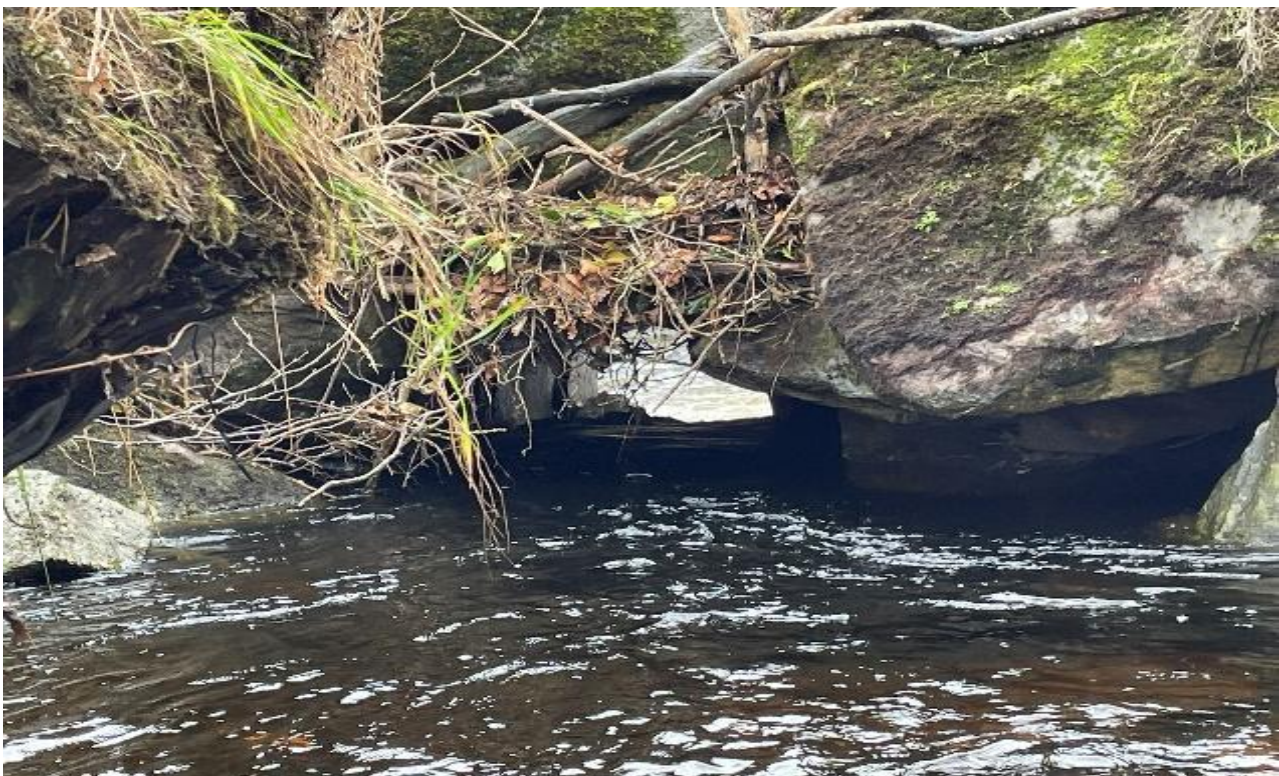
Figure 40: downstream view of the Rough Burn Barrier to fish migration.
