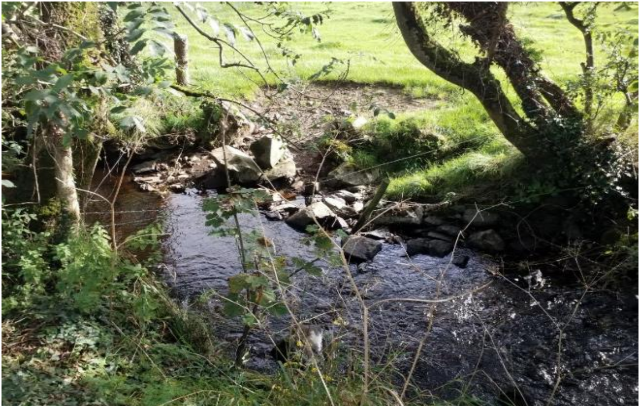
Figure 18: Bank erosion on the Dresnagh from livestock poaching.
