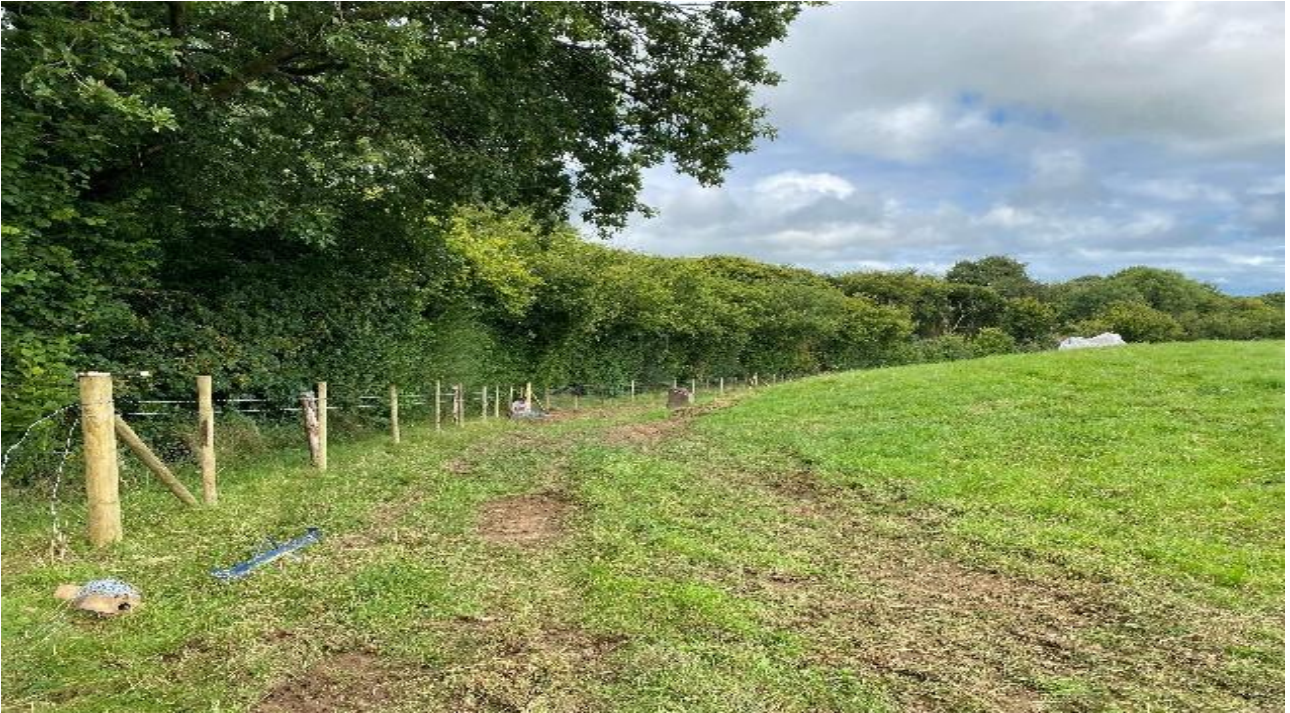
Figure 20: Fencing along the banks of the Dresnagh River.
