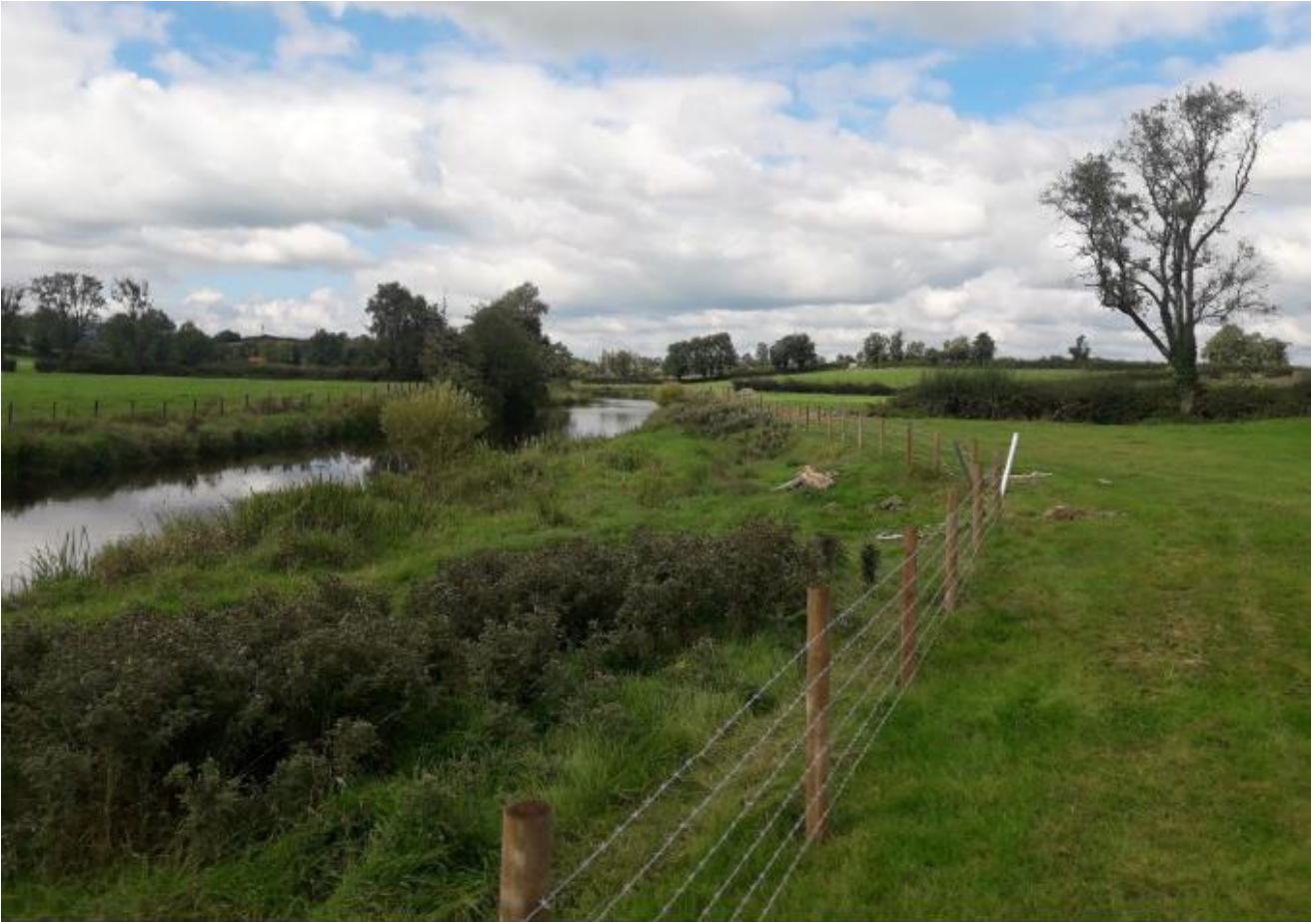
Figure 78: fencing installed to encourage vegetation growth on the banks.
