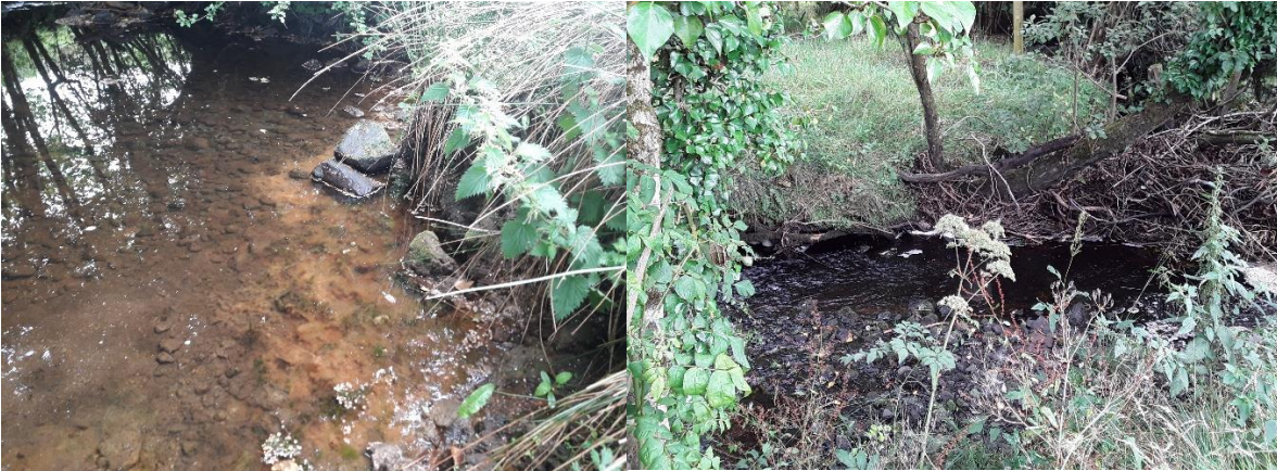
Figure 109. Substrate condition before and after measures.
