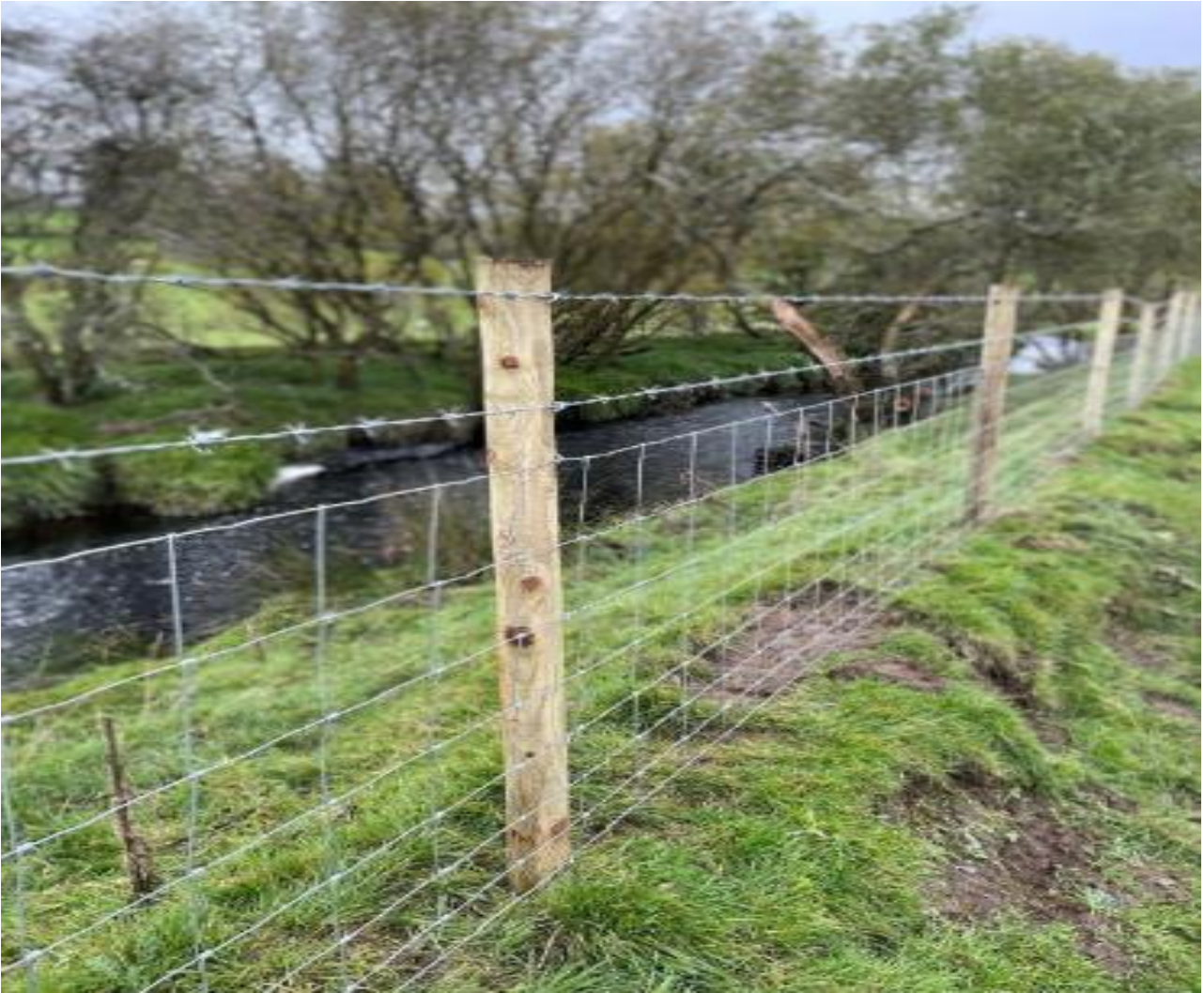
Figure 12: Riparian fencing installed along the Elatagh.
