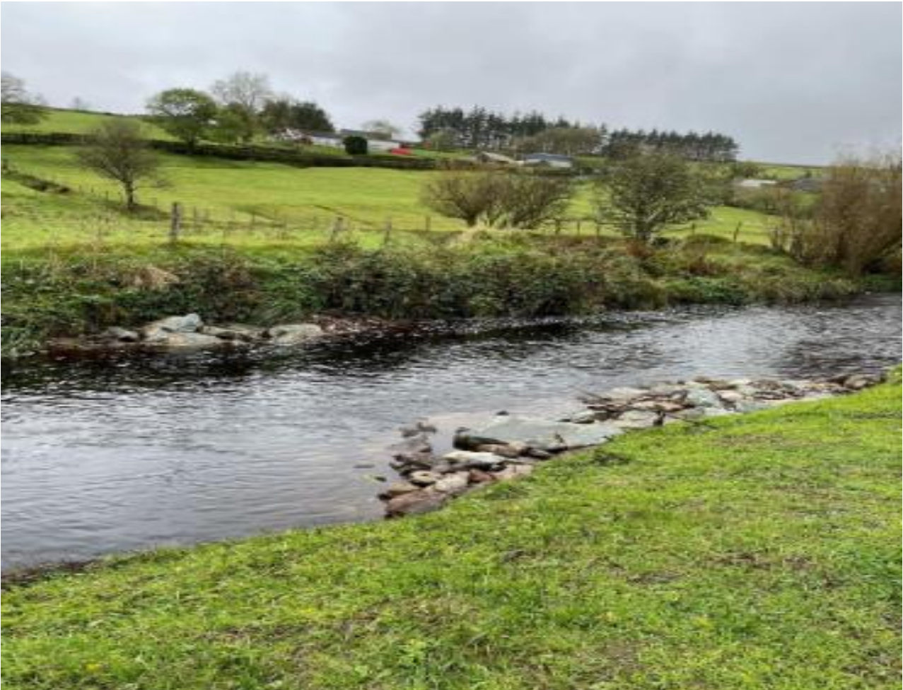
Figure 13: Artificial Meanders complexes installed
