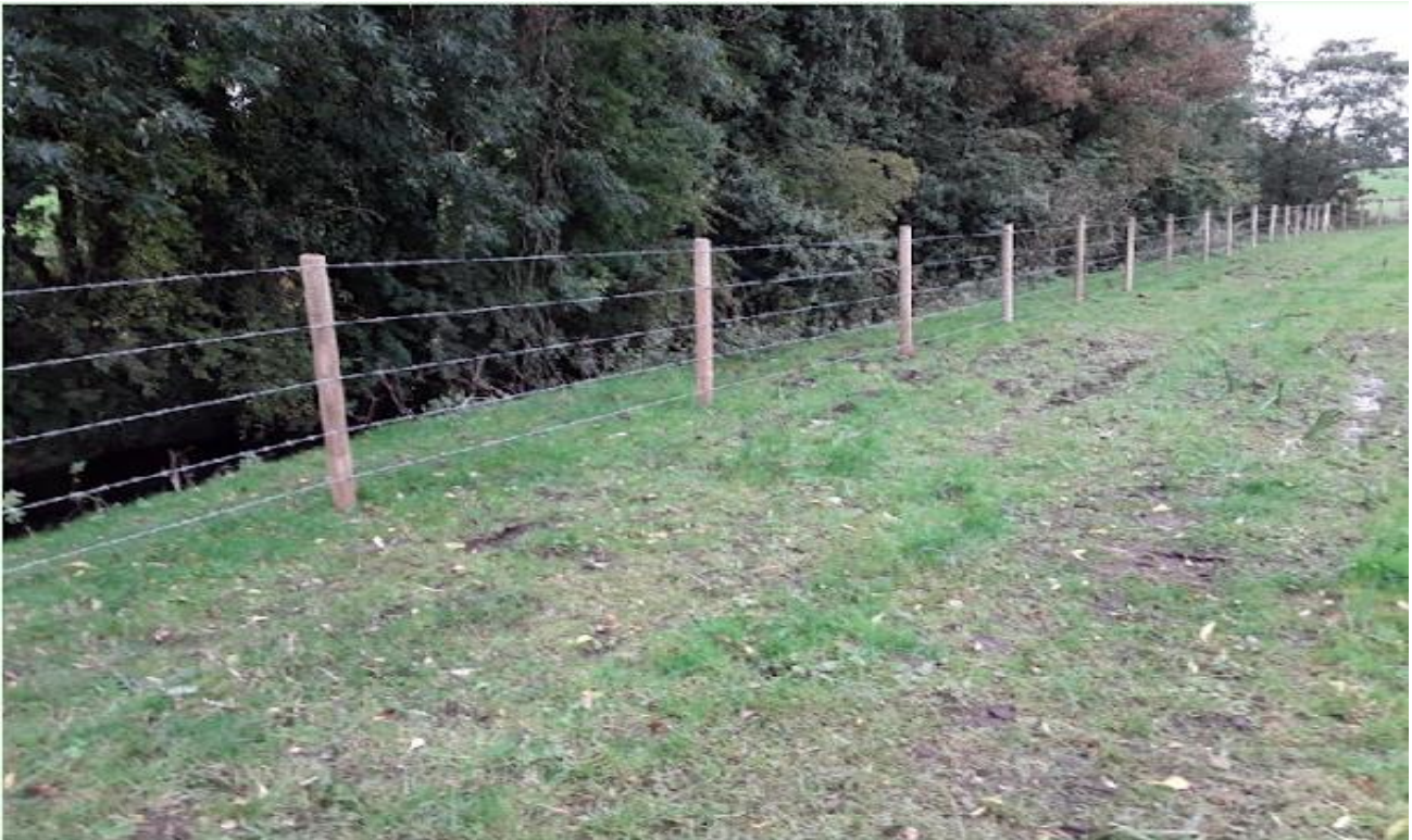
Figure 145: Fencing installed to prevent livestock access to river
