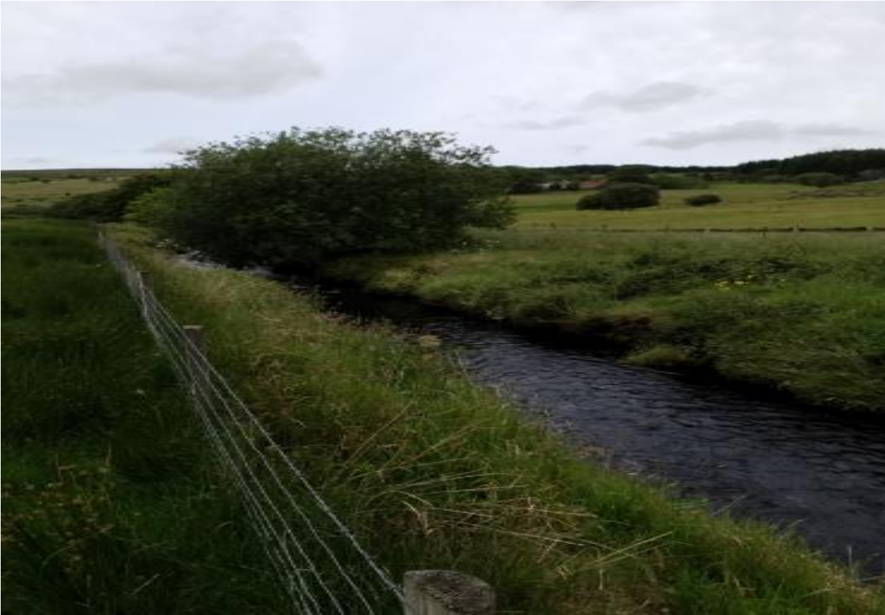
Figure 10: Banks had been fenced off in areas and had lacked appropriate riparian margins.
