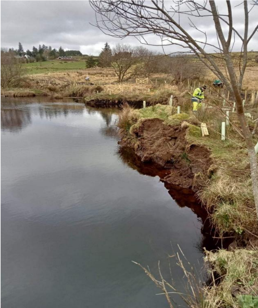
Figure 39: Planting of 900 native broadleaf trees along the Finn 001 stretch to provide adequate riparian margins and improve ecosystem diversity.
