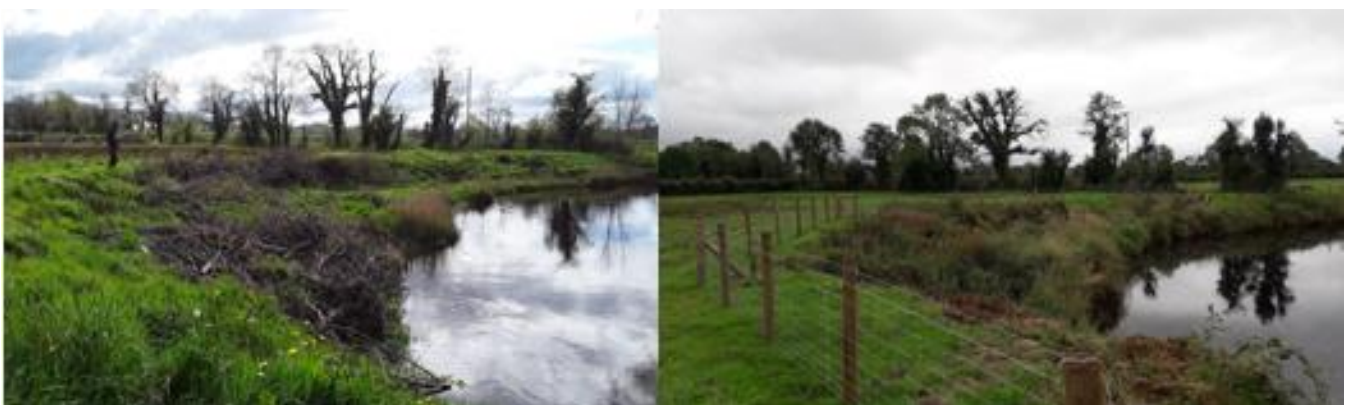
Figure 70: Installation of fencing before and after works.
