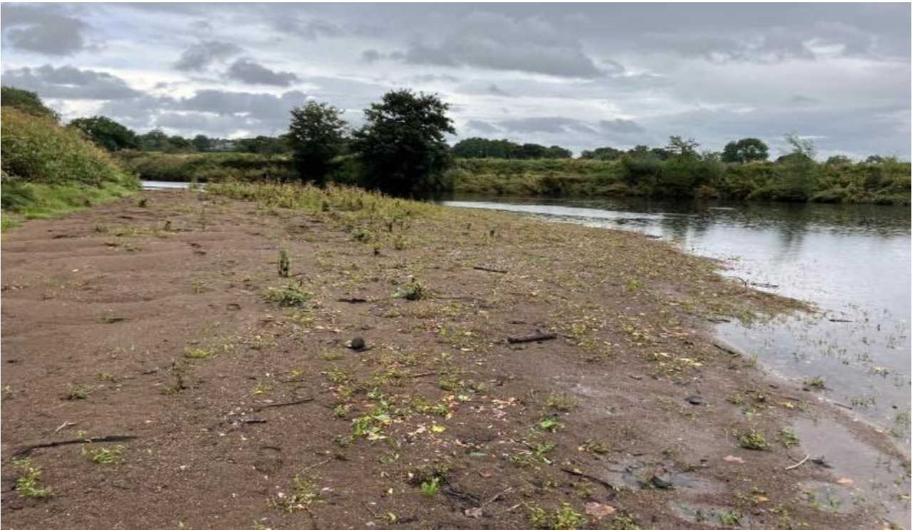
Figure 35: area of high and dry gravel was reggraded into the river to create spawning habitat for salmonids.
