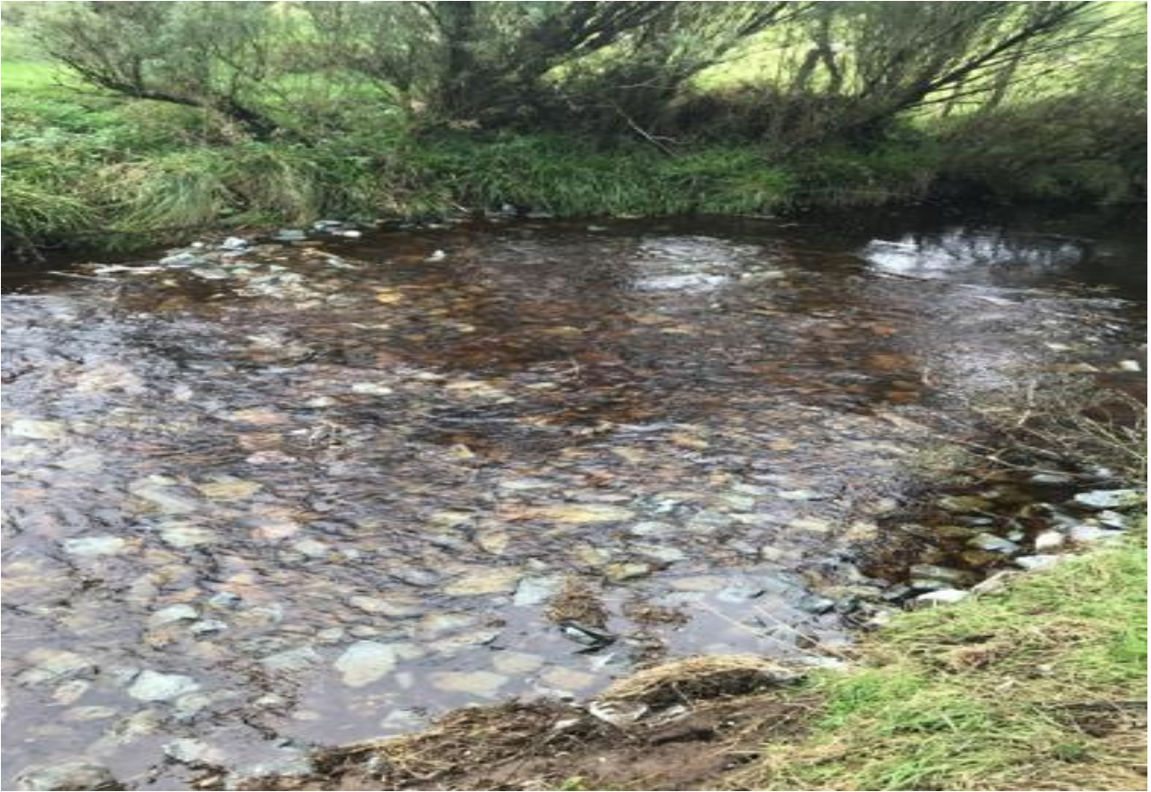
Figure 14: Rubble Mats installed within the Elatagh River.
