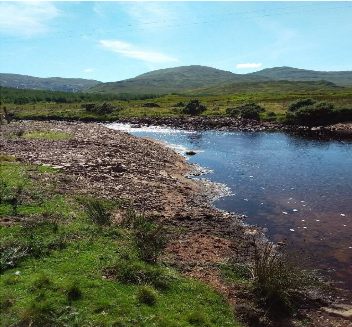
Figure 52: a large bank of high and dry gravel had been regraded into the river to provide spawning habitat for salmonids.
