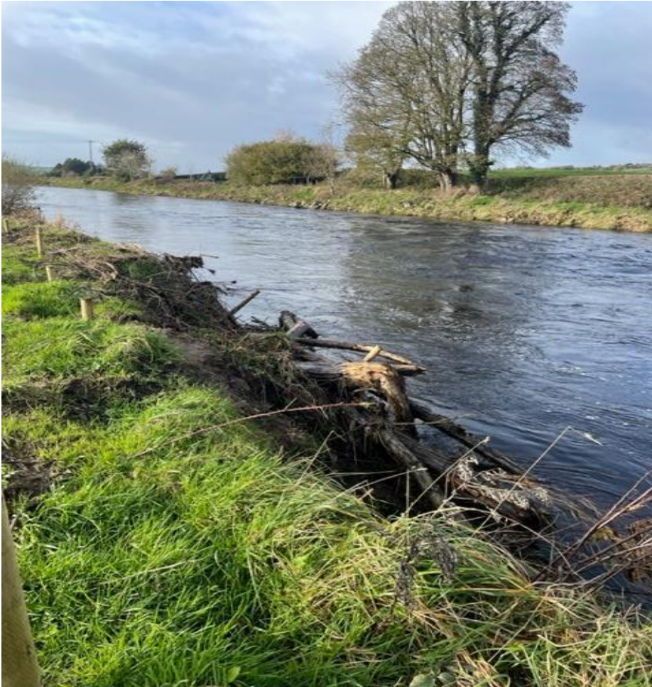
Figure 34: pinned woody material implemented at 6 locations of the Finn 003 stretch.
