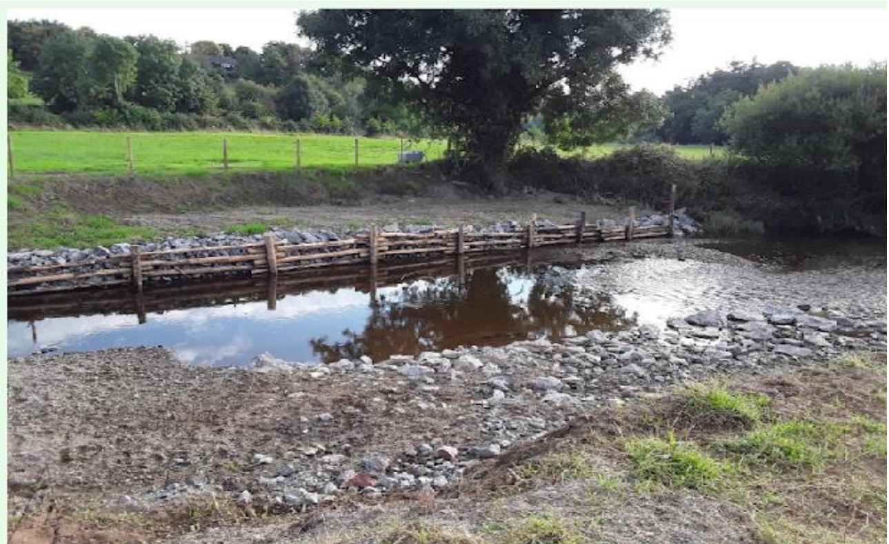
Figure 146: Log wall implemented
