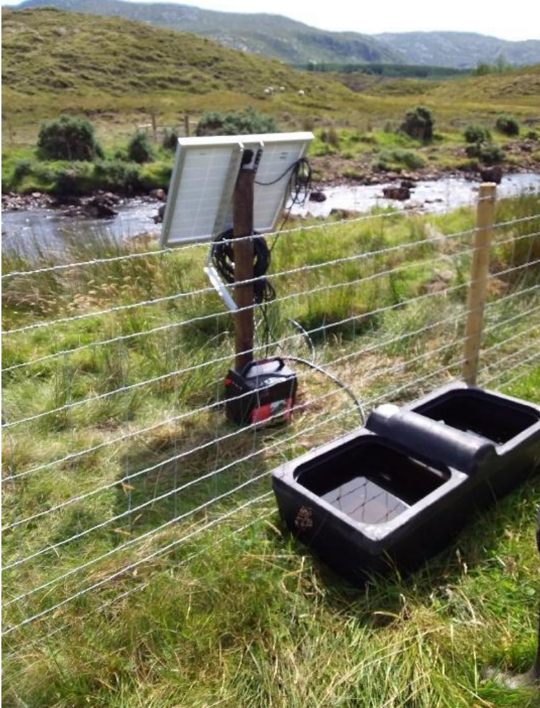
Figure 51: Solar powered pump and trough installed for livestock welfare.
