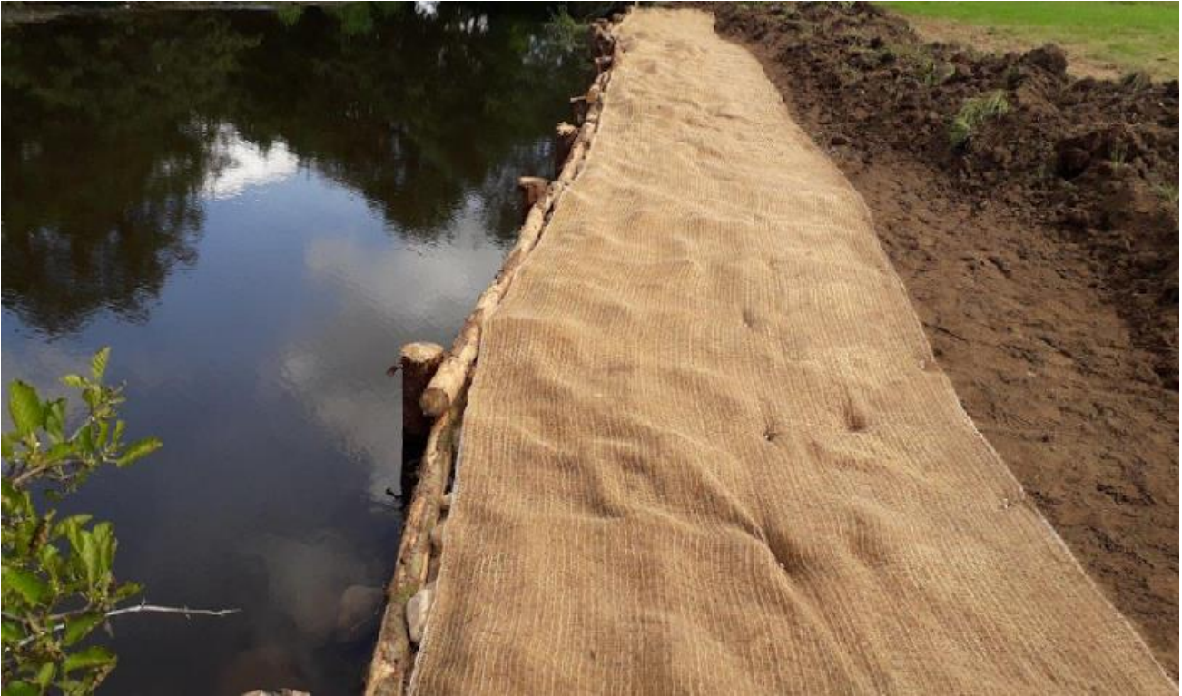
Figure 125: Coir Matting Installed
