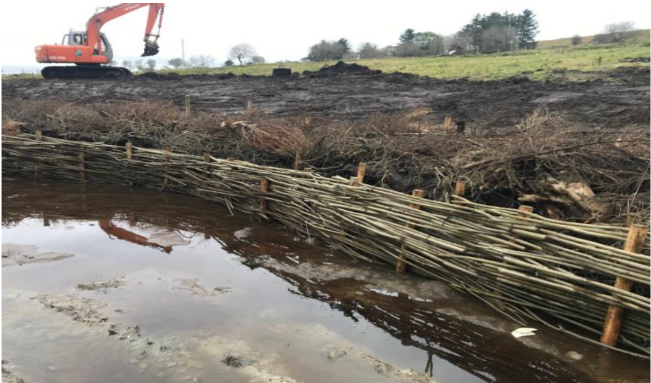
Figure 6: Live Willow weave wall with brash material packed behind.
