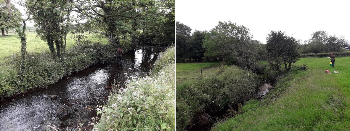
Figure 84. Natural channel morphology (left) and altered over-deepened channel with steep banks (right) 200 m downstream.
