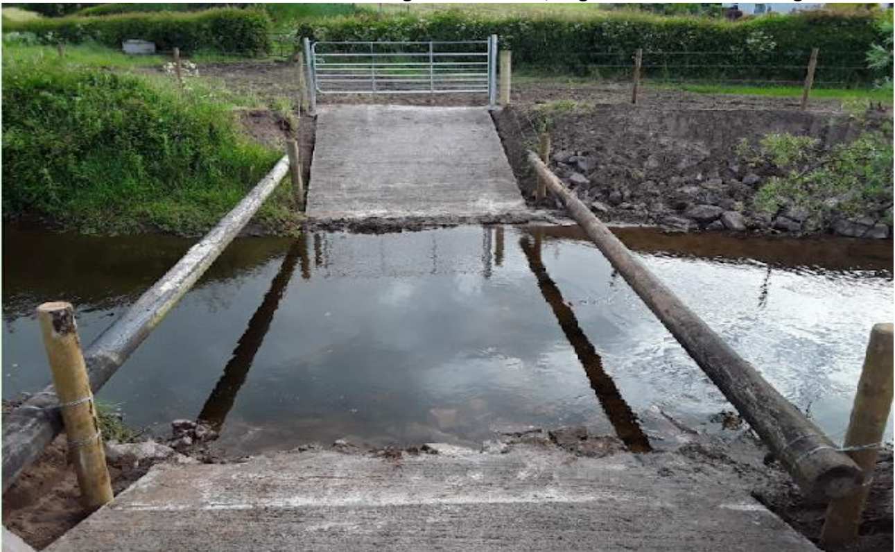
Figure 133: River crossing installed
