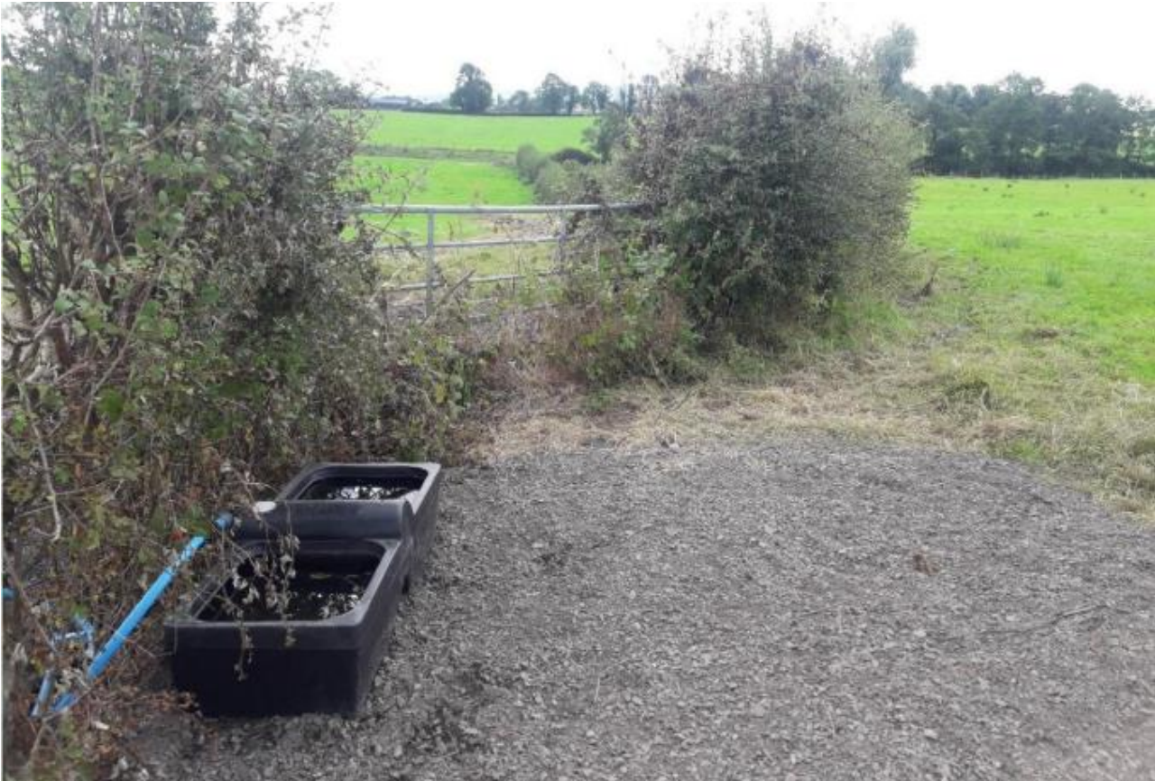
Figure 80: Livestock drinker with hard core installed away from the river to reduce soil exposure and to provide an alternative drinking solution for cattle.
