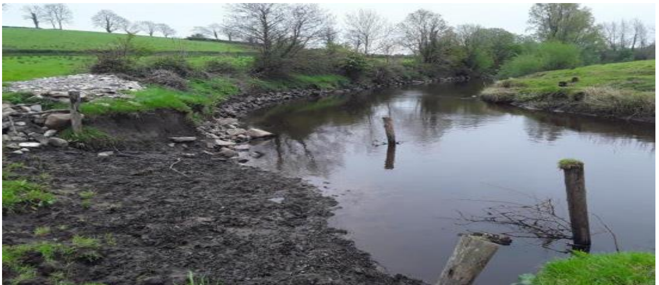
Figure 56: Cattle Poaching with large amounts of sediments with bank toe reinforcement.
