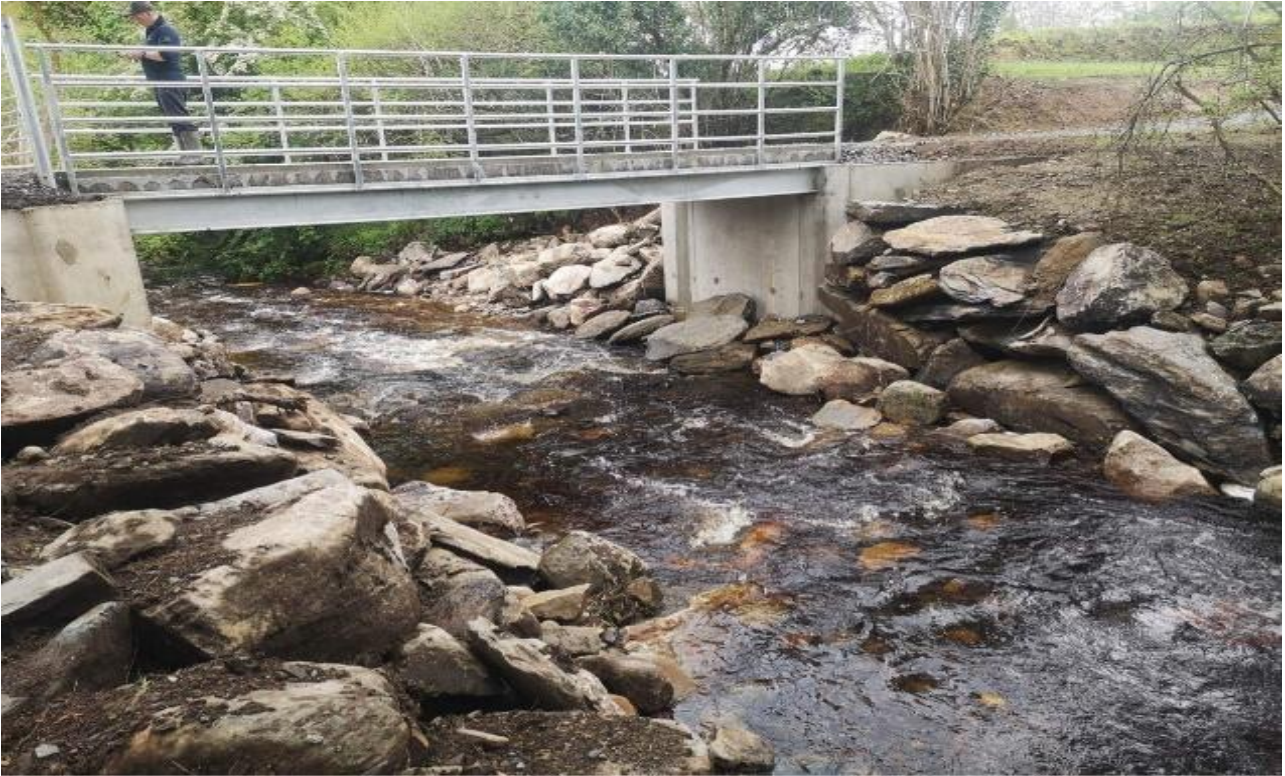
Figure 46: Clear span bridge replaced the prior crossing which was a barrier to fish migration.
