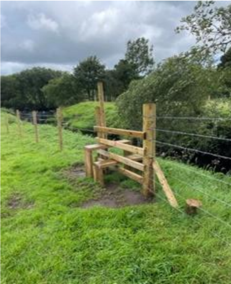
Figure 44: one of the 9 stiles installed along the Rough Burn restoration works for landowner and angler access.
