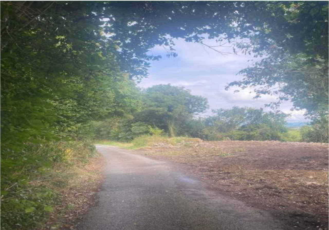
Figure 22: area of land cleared and levelled for recreational walkway for the Community around the Dresnagh River.
