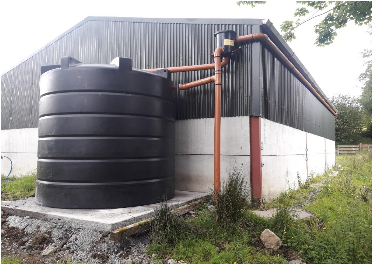
Figure 93. Installation of rainwater harvesting system.
