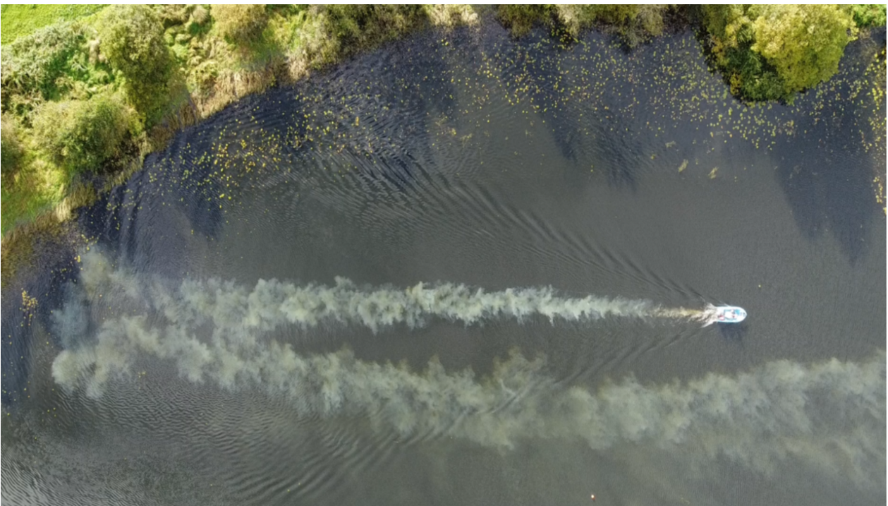
Figure 5 – Grove Lough being dosed with 0.3 tonnes of Alum on 19/10/2021. Note the floc plume precipitating out as alum is mixed into the water column by the boat propellor. When dispensing the chemical salts, the boat travelled in sweeps 7-8m apart, across the long axis and then short axis in a grid pattern. In this way the chemical is dispersed most evenly throughout the lake water column.
